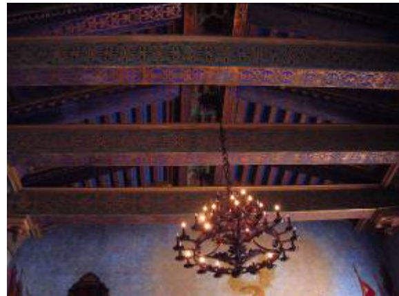
Detail of ceiling in the court chamber
